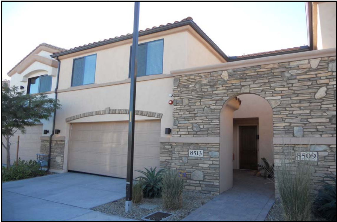
Looking at front elevation of typical subject unit
